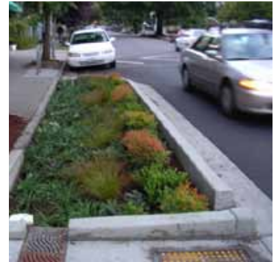
An urban infiltration planter with decorative trench grate.
